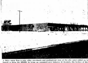
A hill view from a year after construction and production from the city were rolled on to launch a drive for $5,000,000 to bring an unnamed new industry to Oneonta, the factory of Enterprise Aluminum Co. has been completed, and is already ready to start construction of that firm's well-known line of kitchenware. (Star Staff Photo.)
