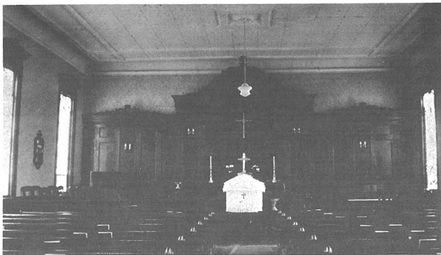
Interior of Methodist Church before renovation
