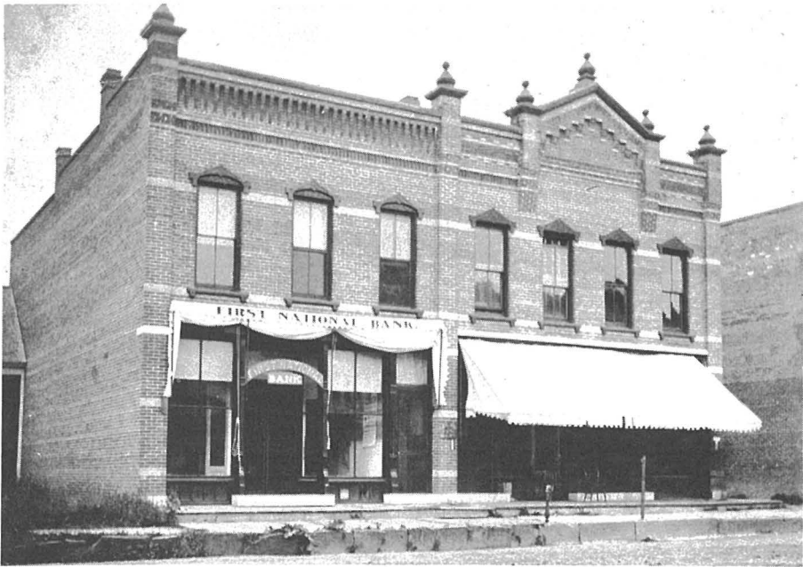
Brick party-building constructed after fire
