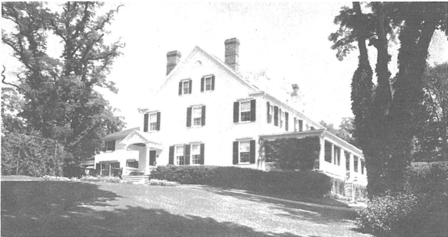
Morris Manor after renovation
