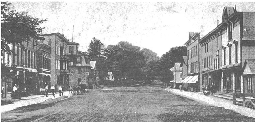
Main Street looking east from Silver Creek bridge
