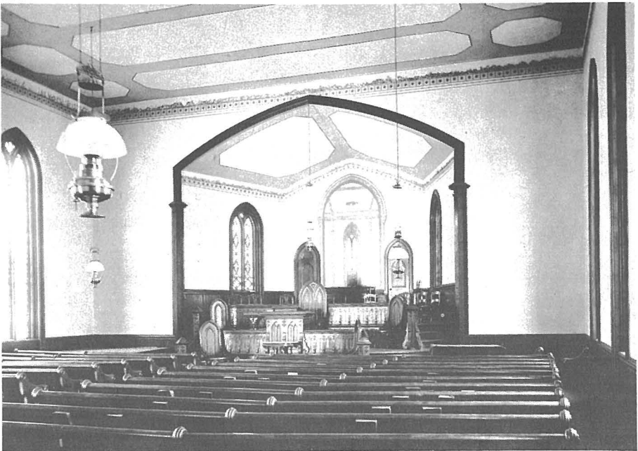
Interior of Baptist Church before renovation
