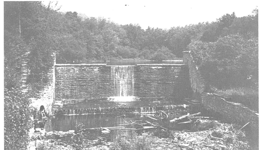
The Dam at Morris Manor
