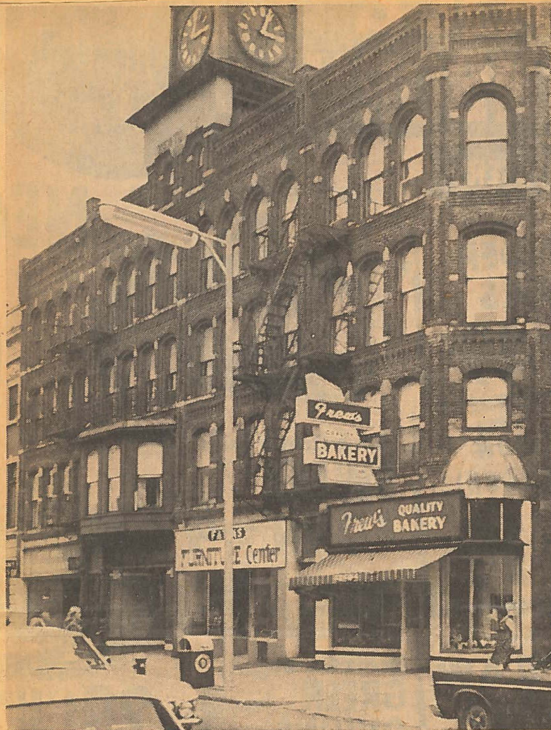
CITY PROPERTY — The Westcott Block on Main Street, one of two pieces of property which have been purchased by the city to be demolished to make way for more downtown parking. The other building, at the rear of the Westcott Block, faces Hamilton Avenue and currently houses the Daley plumbing shop. (Star staff photo)
